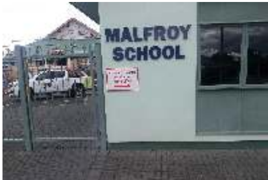
Side entrance next to staffroom
